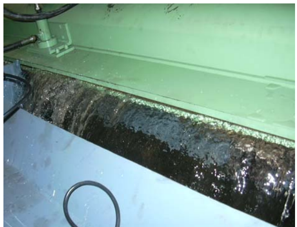
Figure.9 Water curtain cooling system
